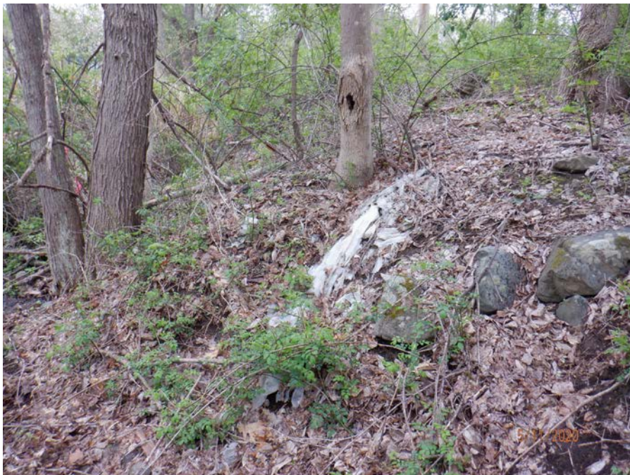
Photograph 8: Impact Area 2 – Buried plastic in old fill, tree cavity in background.
