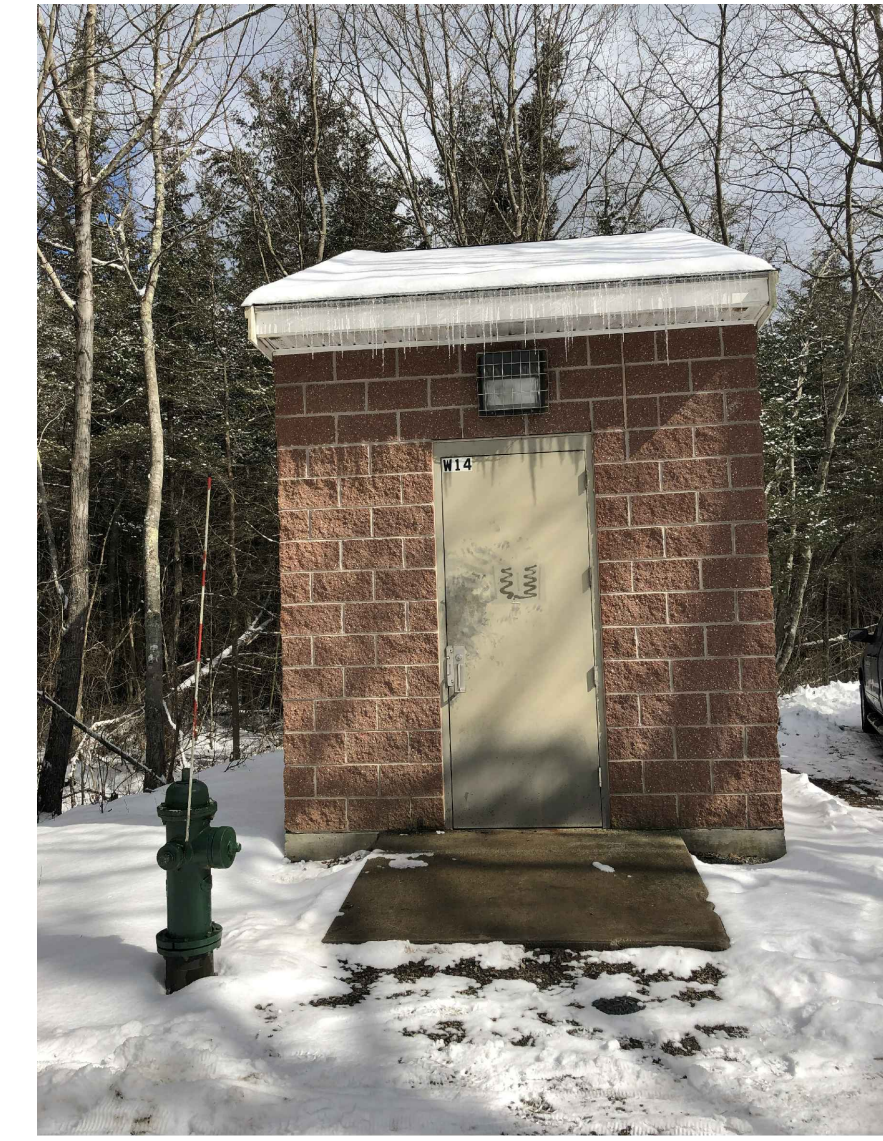
PHOTO 2 SCALE: N.T.S. WELL STATION 14 LOOKING EAST
