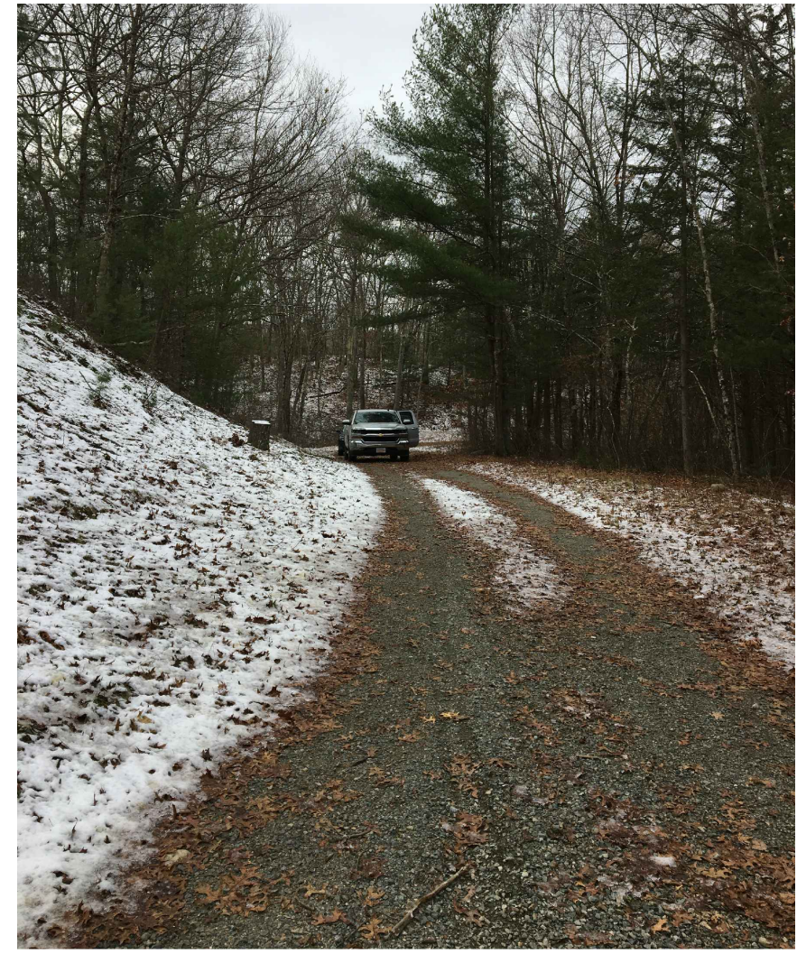
PHOTO 3 SCALE: N.T.S. GRAVEL ACCESS DRIVEWAY LOOKING WEST
