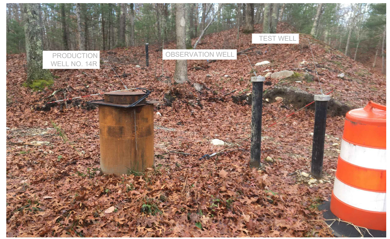
PHOTO 1 SCALE: N.T.S. OBSERVATION WELL, TEST WELL, AND PRODUCTION WELL NO. 14R LOOKING SOUTHWEST
