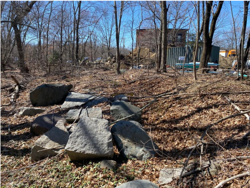
Photo 2: Disturbed Buffer Zone and BLSF behind container and piles, 3/30/21
