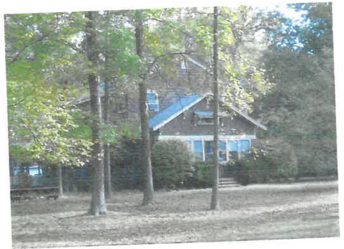
abutting property to north
