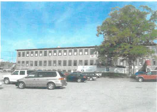
former mill to southwest
