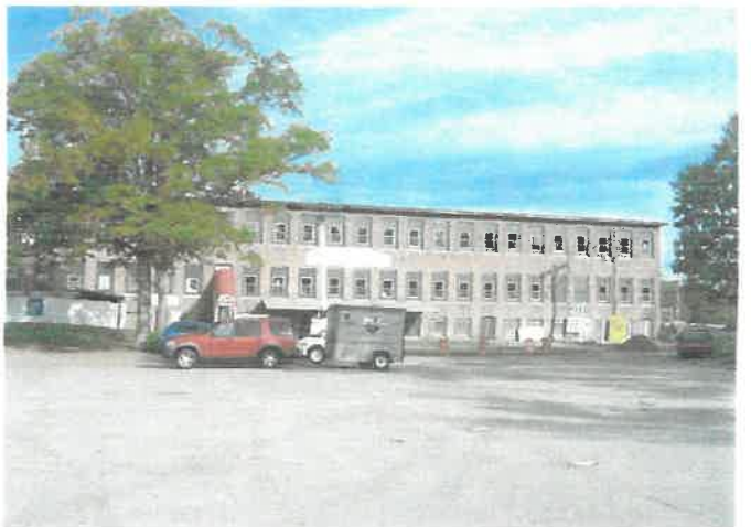
former mill to southwest
