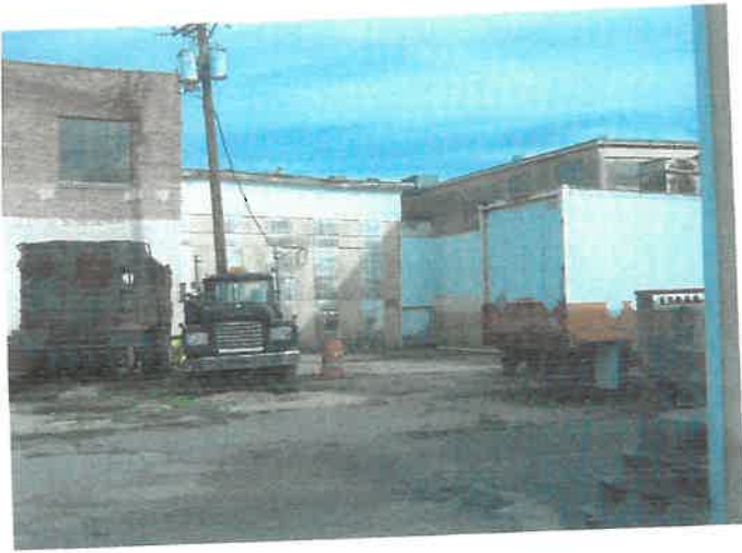
former mill to southwest
