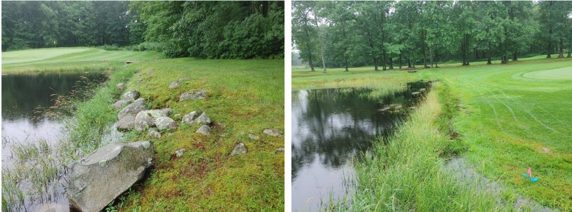
Left Photograph: View facing east of existing stone-lined portion of Bank. July 2, 2021.
