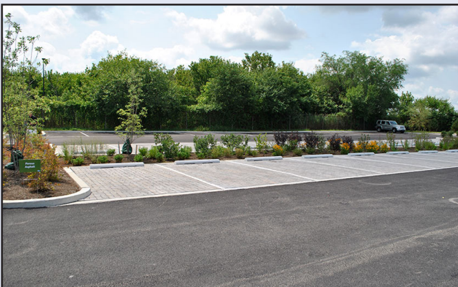
Parking ROW Bioretention
