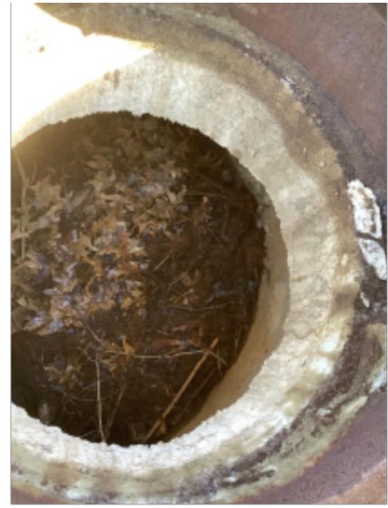
MH Upstream from outfall
