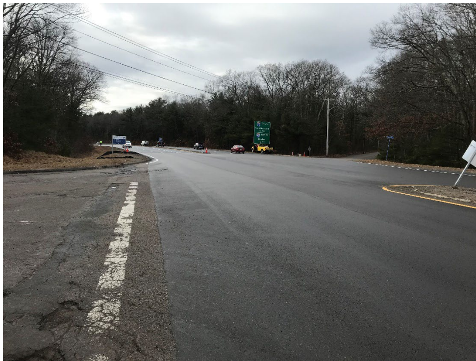
Figure 3 –Commercial Street & Walnut Street intersection. Photo taken facing southwest.
