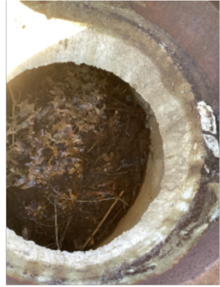
MH Upstream from outfall
