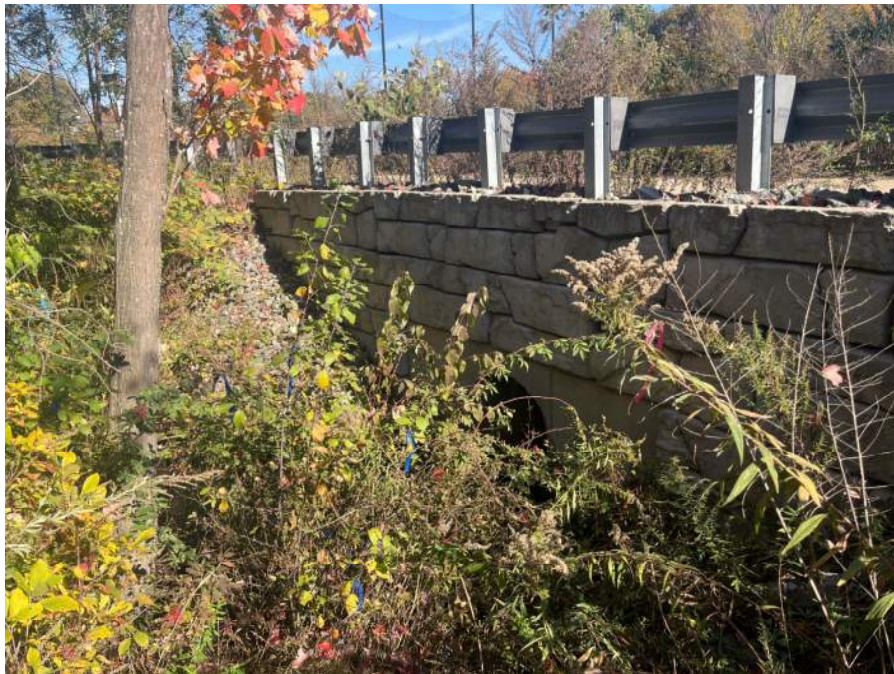
Photo 2: Recently replaced culvert passing R-series stream beneath access road.
