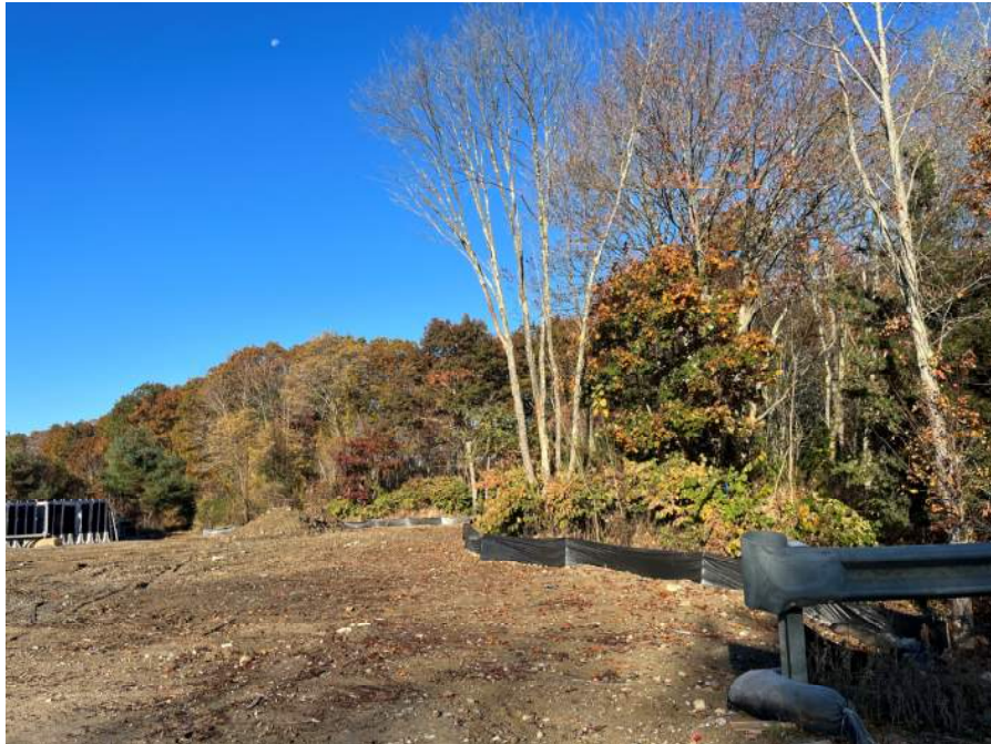
Photo 14: Eastern portion of prepared site. Silt fence along treeline has recently been replaced.
