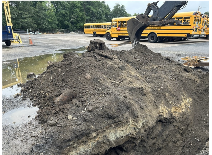
2. Excavated Soil Profile
