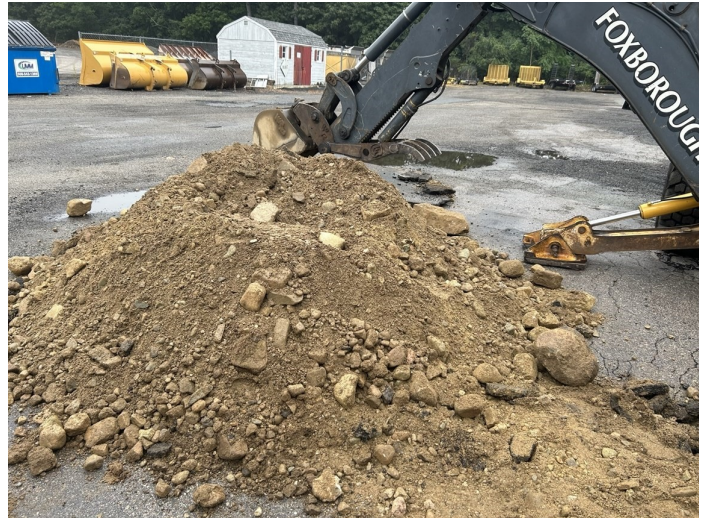
2. Excavated Soil Pile
