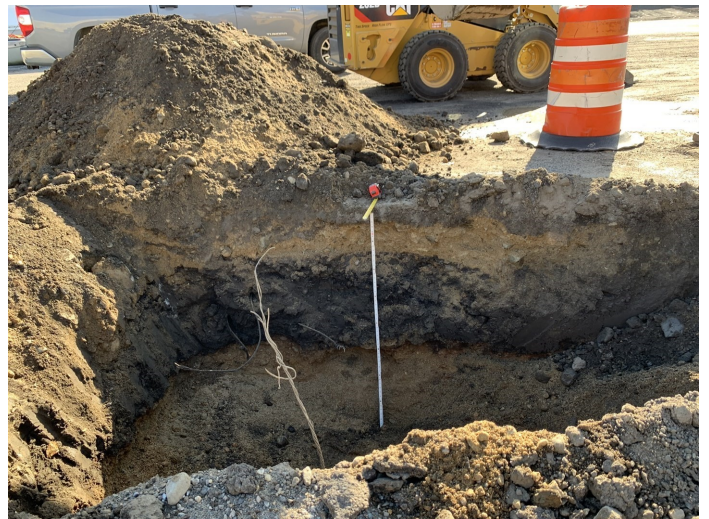
TP-101 - Sidewall View 2
