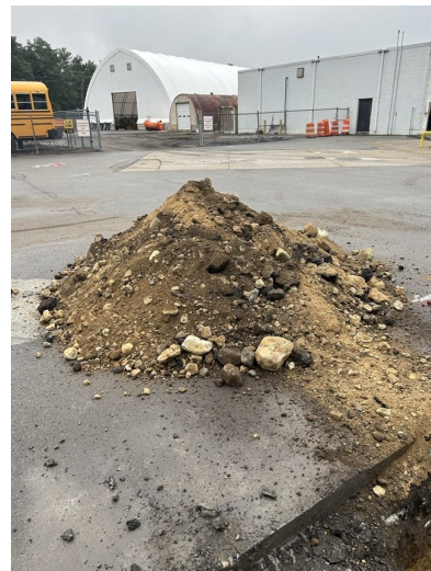
2. Excavated Soil Pile
