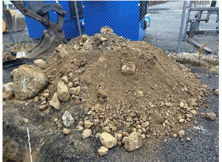
2. Excavated Soil Pile
