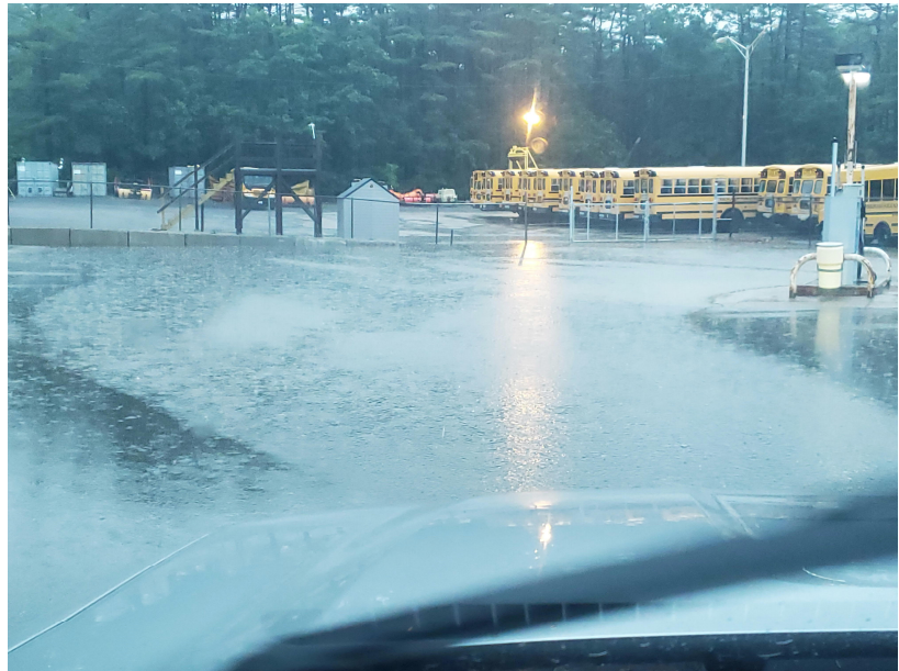
Flooding at the Highway Garage
