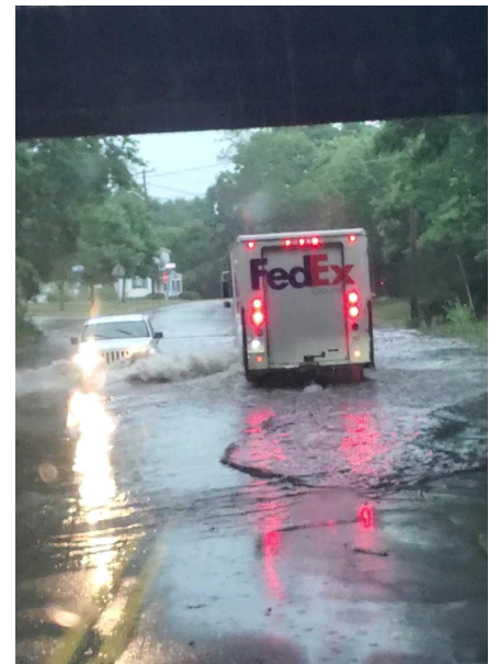
Flooding at the Cocasset St. rail underpass
