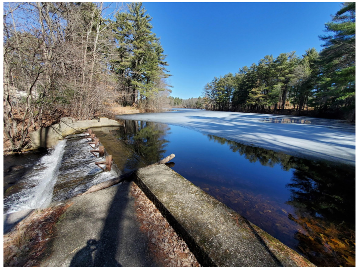
Foundry Pond Dam
