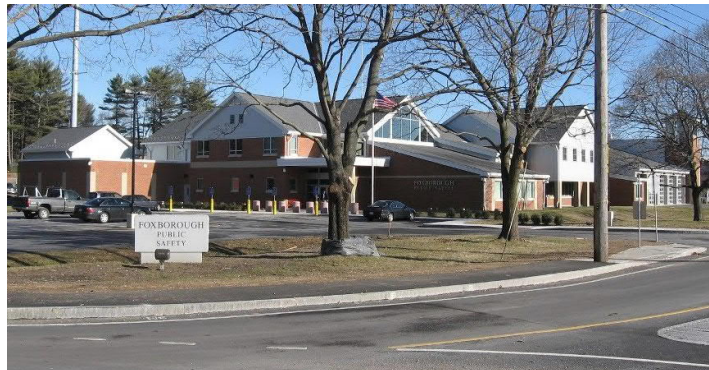
Foxborough Public Safety Complex
